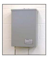
The **STAR**® DCU is mounted in a convenient location such as a utility closet or storage room. The DCU contains a radio receiver, computer, and a modem. Power is provided by a 120 vac source.
